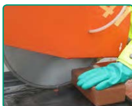
Cutting engineered brick.
